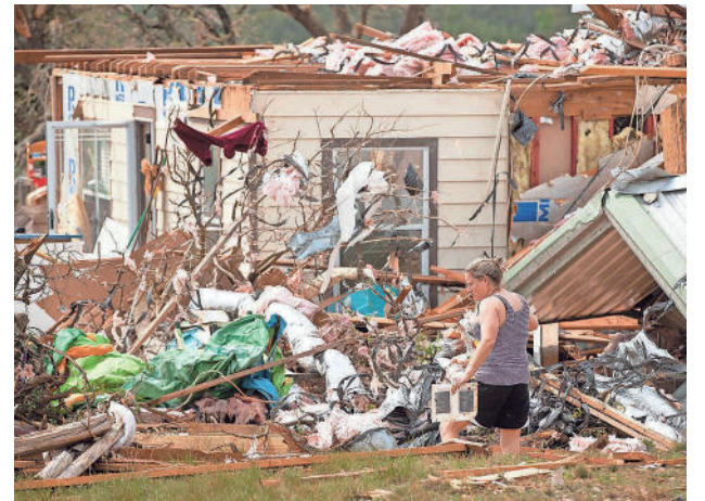
Michelle Light salvages belongings from her home at FM 2843 and Cedar Valley Road near Salado a day after a tornado destroyed the house last April.
